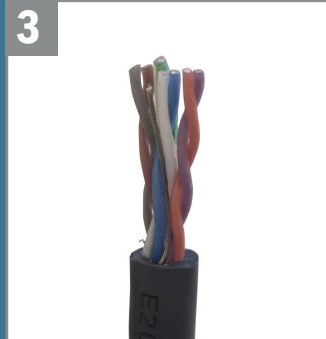
3 Strip 1" of jacket. Leave the uninsulated ground wire for now.
