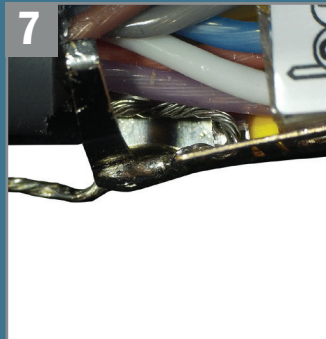
7 Solder drain wire (bare wire to connector body). Trim excess tail wire.
